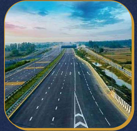
250 M WIDE 6 LANE EXPRESS HIGHWAY AHMEDABAD-DHOLERA
