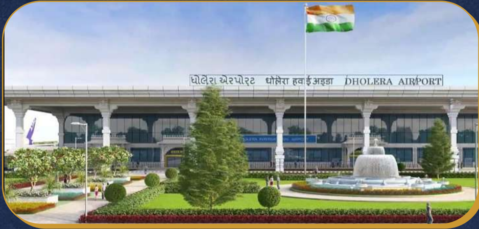
DHOLERA INTERNATIONAL AIRPORT
