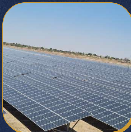
WORLD'S LARGEST SOLAR PARK (5000 MW)
