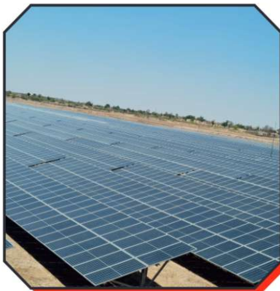
WORLD'S LARGEST SOLAR PARK (5000 MW)
