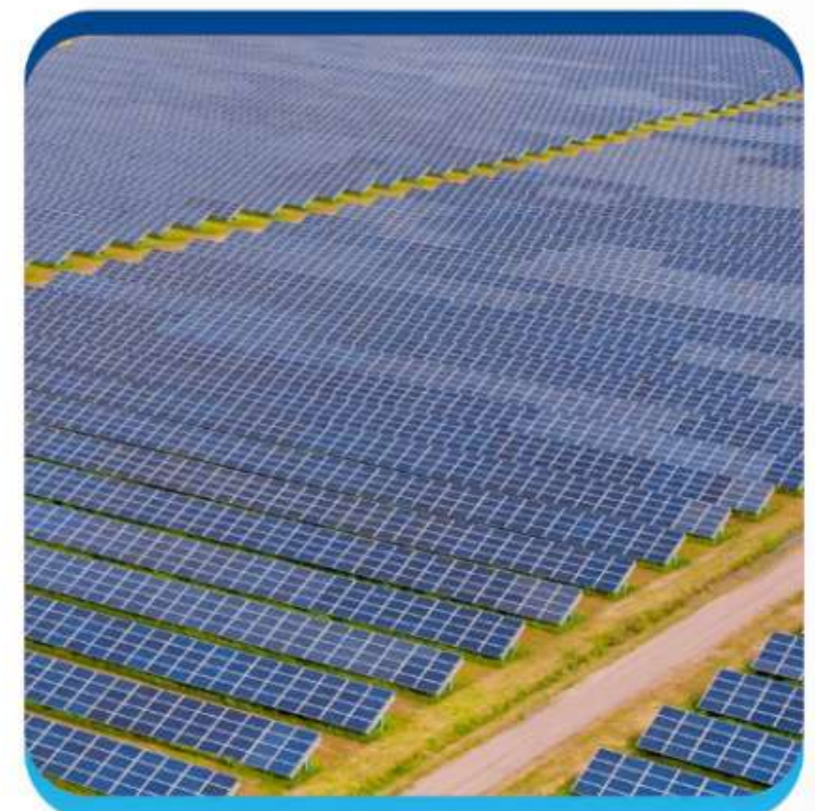
WORLD'S LARGEST SOLAR PARK (5000 MW)
