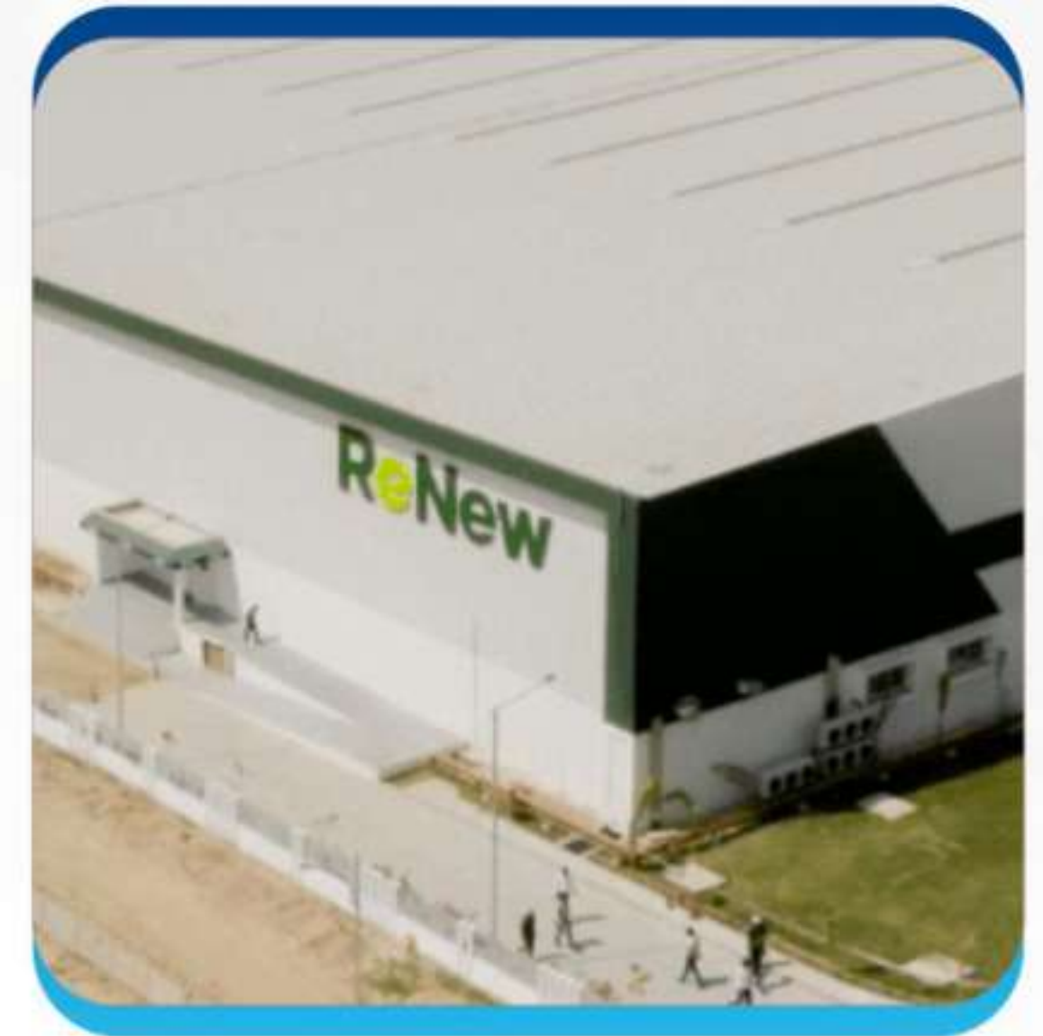
RENEW POWER-2000MW SOLAR CELL 1200 CR CONSTRUCTION COST
