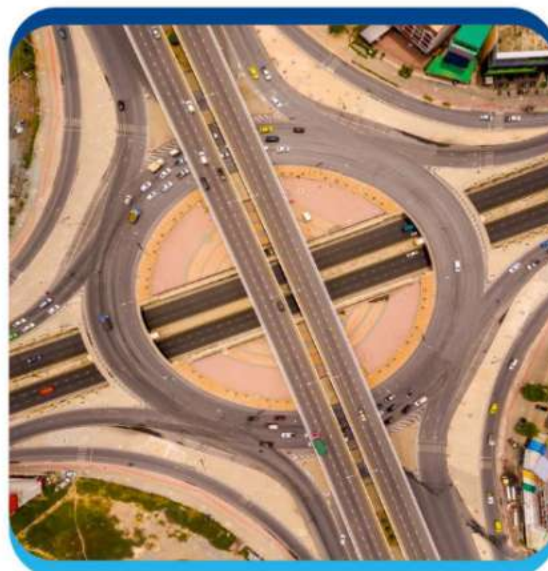
250 M WIDE 6 LANE EXPRESS HIGHWAY AHMEDABAD-DHOLERA
