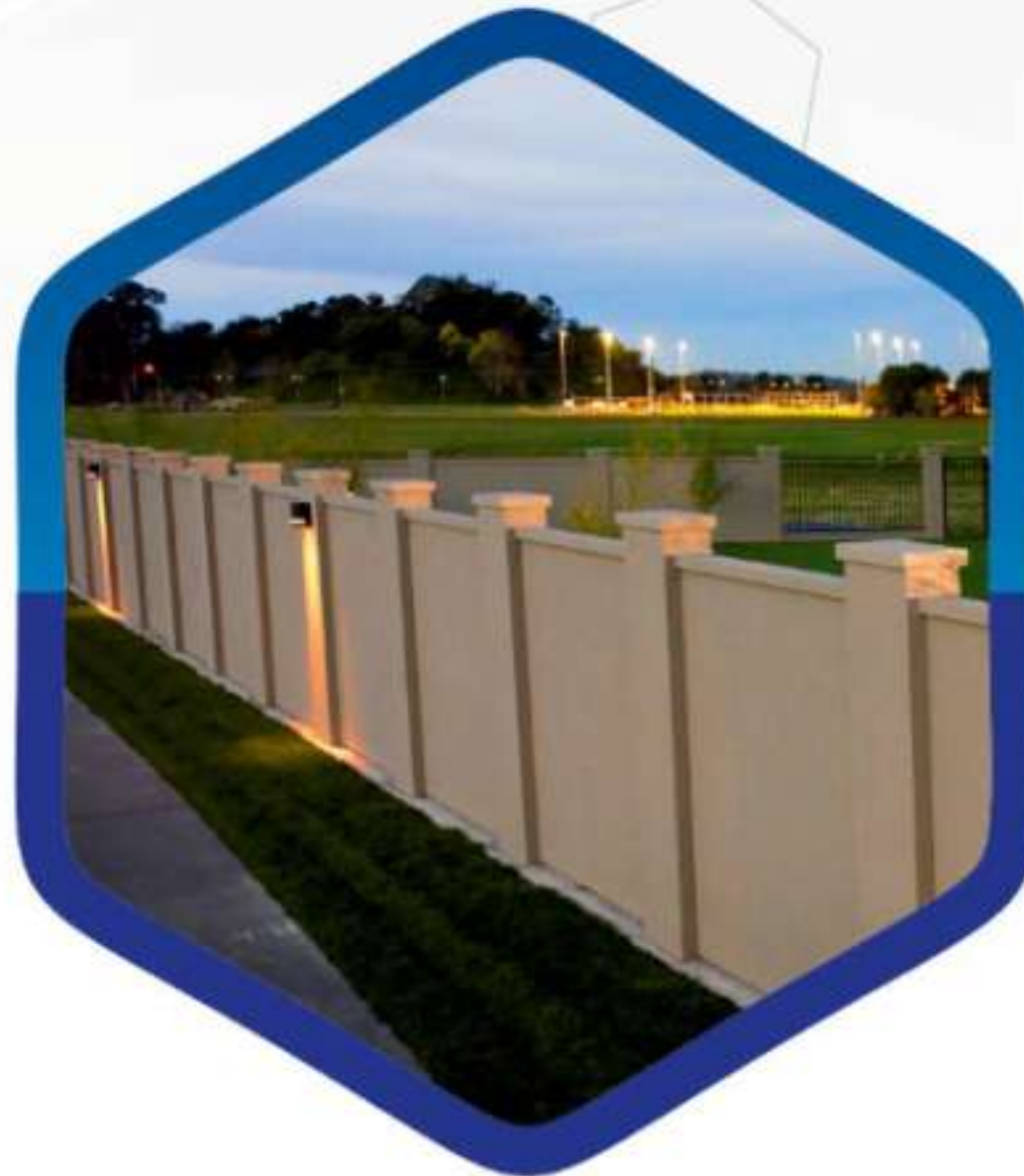
PROJECT BOUNDARY (COMPOUND WALL)
