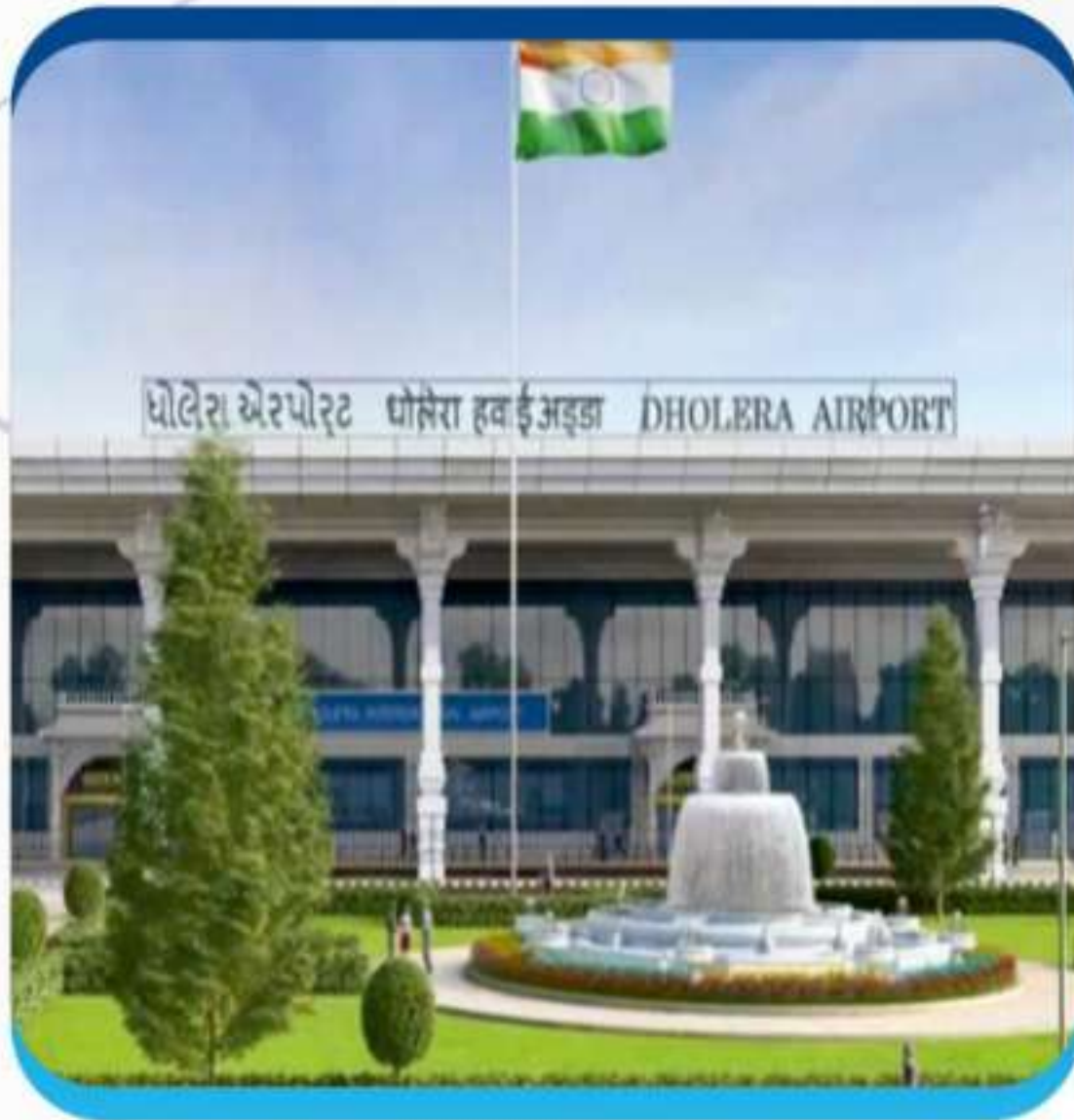
DHOLERA INTERNATIONAL AIRPORT
