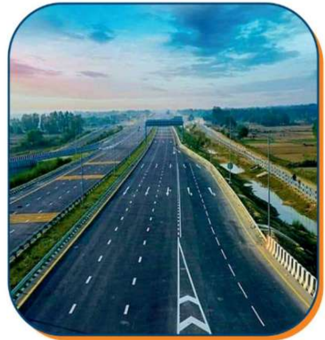
250 M WIDE 6 LANE EXPRESS HIGHWAY AHMEDABAD-DHOLERA
