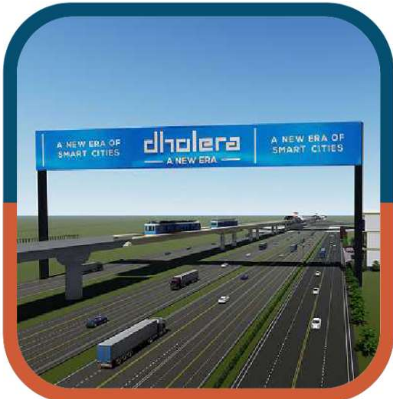
250 M Wide 6 Lane Express Highway Ahmedabad-dholera
