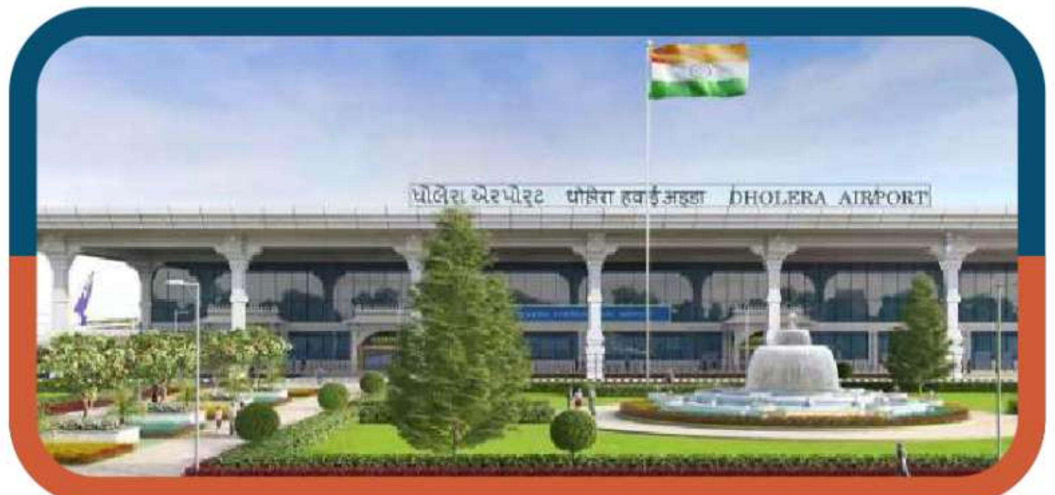
Dholera International Airport
