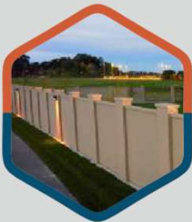
PROJECT BOUNDARY (COMPOUND WALL)
