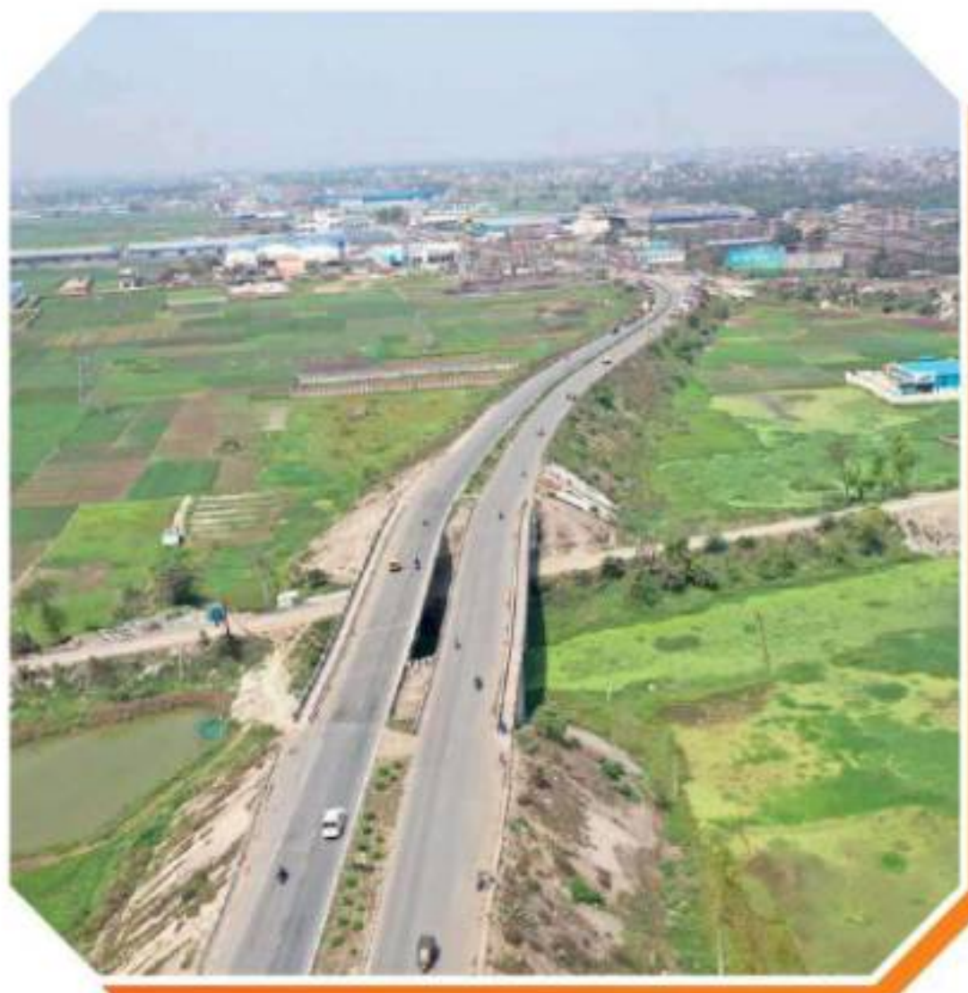
250 M WIDE 6 LANE EXPRESS HIGHWAY AHMEDABAD-DHOLERA
